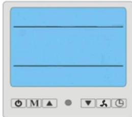
Picture: Blank display indicates no power supply and complete shutdown of the heat pump.
