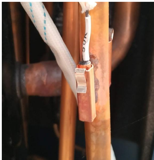
T4 – Compressor discharge temperature
