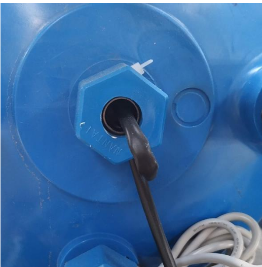
T5 – Outlet water temperature
