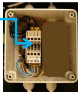
Picture: Four pin terminal connection of water unit (1-4 sensor connection with condensing unit).
