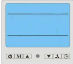
Picture: Blank display indicates no power supply and complete shutdown of the heat pump.
