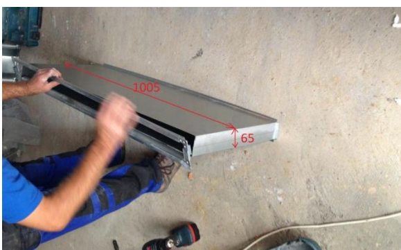
5. Dehumidifier cover assembly
