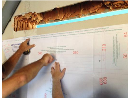
2. Console measuring using template
