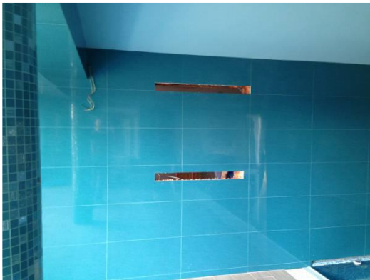
1. Cutting wall transitions
