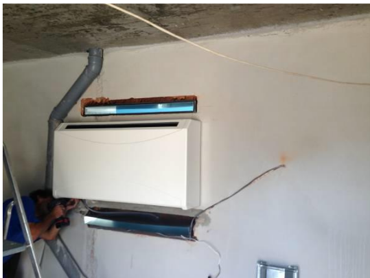
5. Dehumidifier cover assembly
