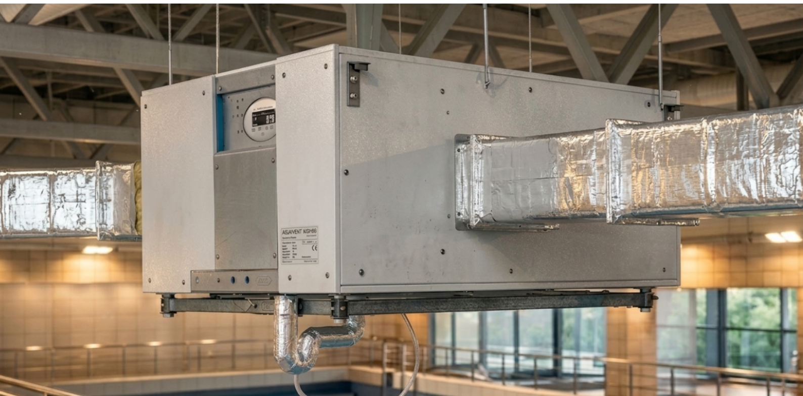
GoldFin protection of air exchanger fins to withstand chlorine and salt
