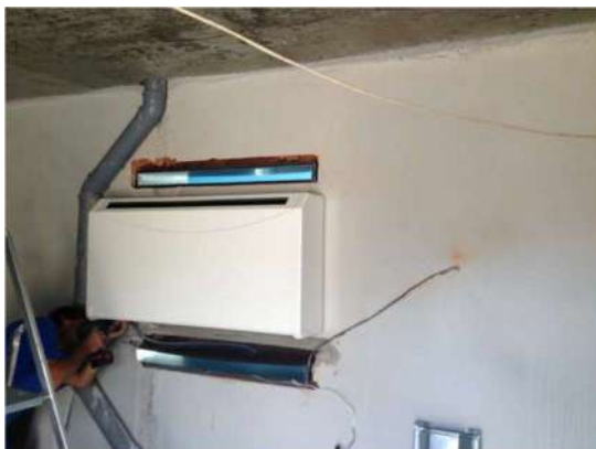
5. Dehumidifier cover assembly
