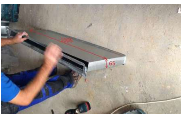
5. Dehumidifier cover assembly
