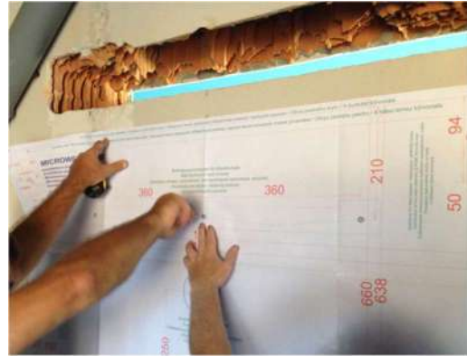
2. Console measuring using template
