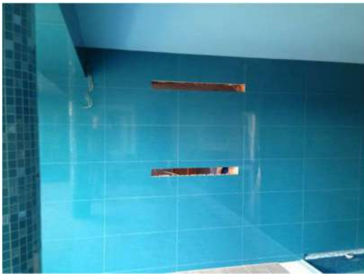
1. Cutting wall transitions
