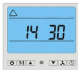
Picture: Parameters check, input water temperature 30°C.
