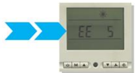
Error code ,EE5' advising of low / high water flow or damaged flow switch.
